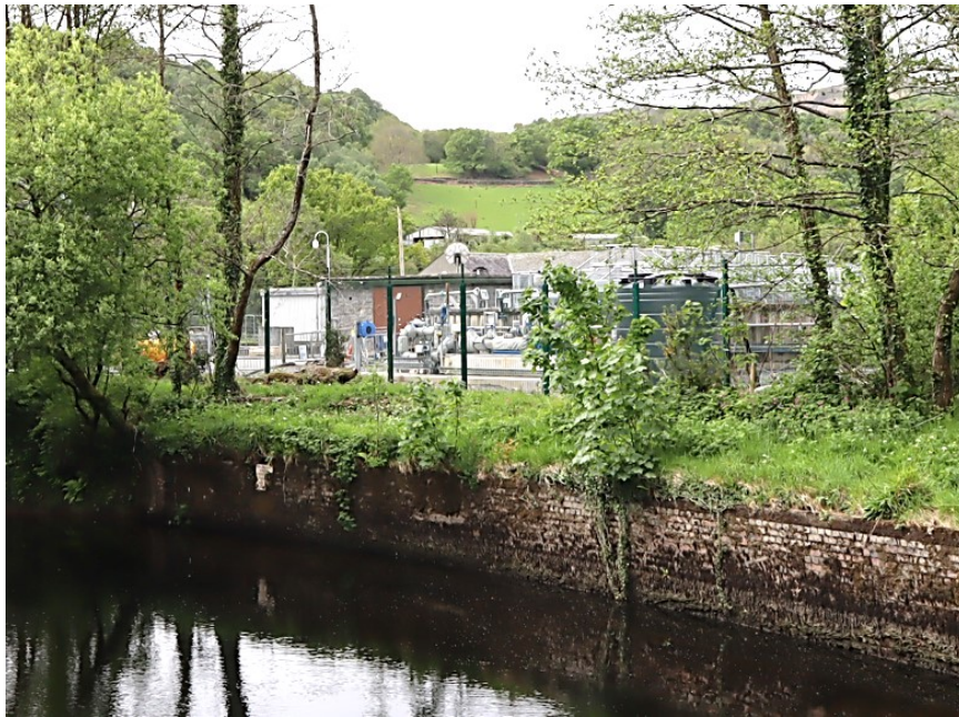
Figure 8: Sewage treatment plant, Dolgellau.
